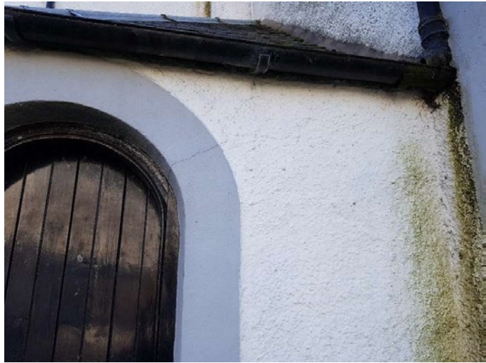
North Elevation Boiler House: Cracks in door margin and harling above. Defective gutter staining wall below.
