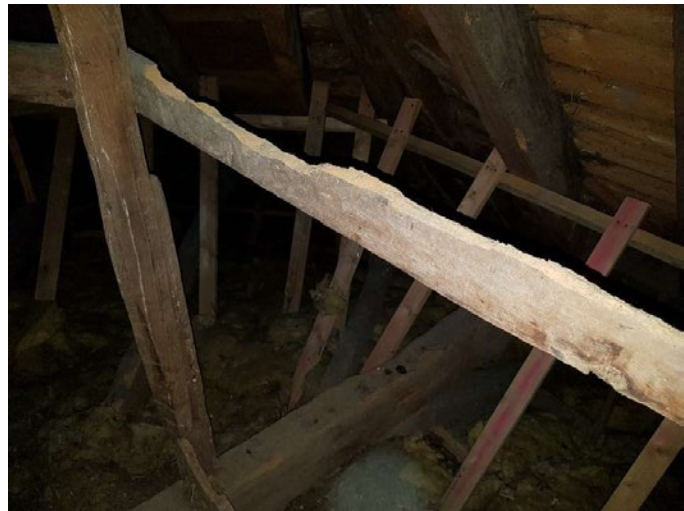
Roofspace: Deterioration to roof timbers from insect attack.
