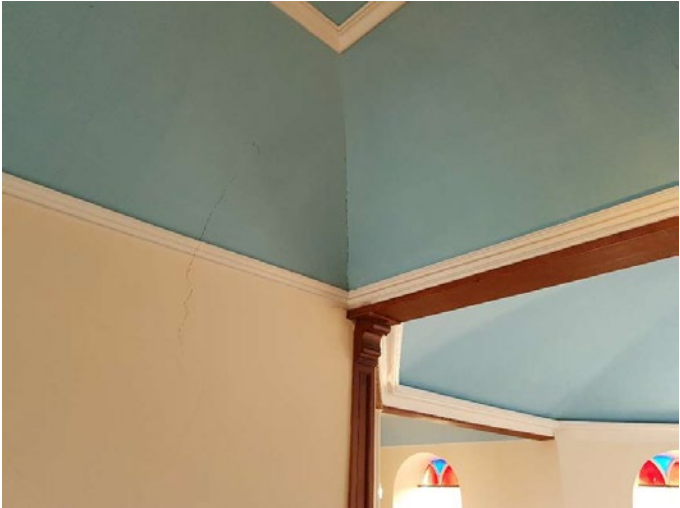
Gallery: Vertical cracking to plaster and cornice.
