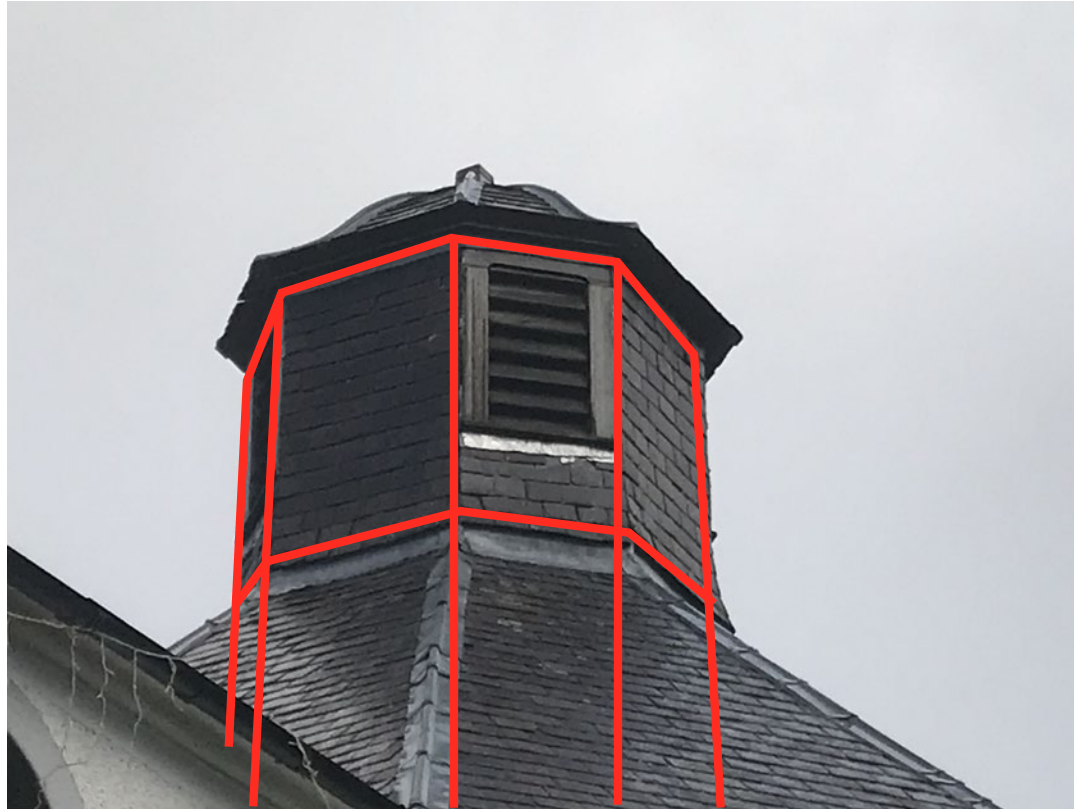
Configuration of the original oak structure, which is carried on the principal roof truss collars.
