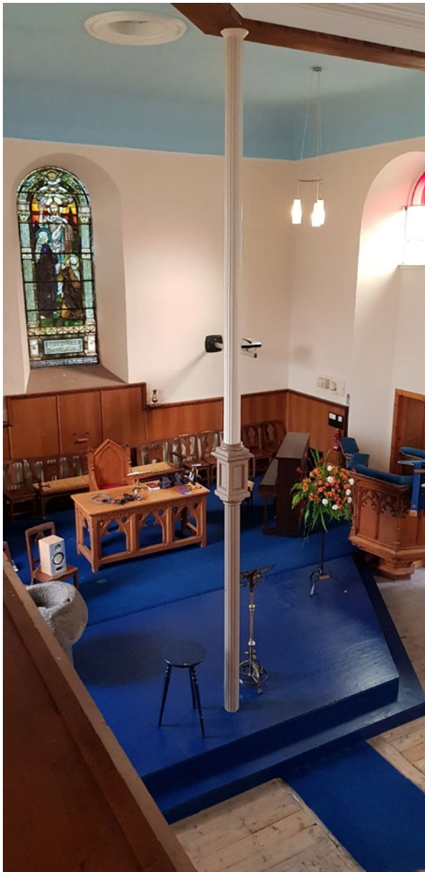
Photograph 4 – Slender cast iron column supporting corner of original octagonal roof above. The circular access hatch into the east roof space can be seen in the adjacent ceiling.
