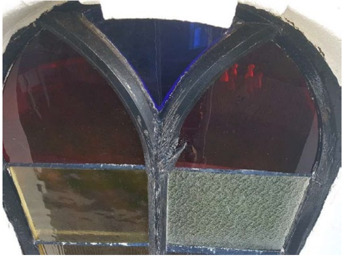
Windows: Defective timber at 'Y' intersection. Different styles and colours of glass used for previous repairs (clear white glass assumed not to be a later replacement).
