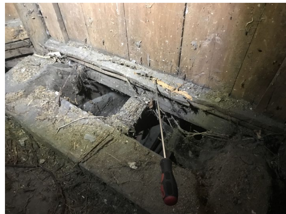
Woodworm degraded softwood plates above unaffected oak frames.
