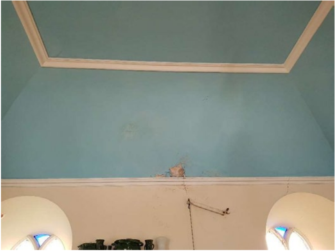
Gallery Ceiling: Cracking to plaster and flaking of paint to ceiling and wall finishes.
