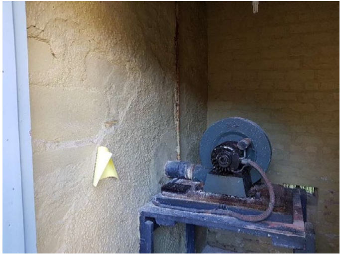
North Elevation Lean-to: Organ blower machine. Evidence of earlier harl on walls.
