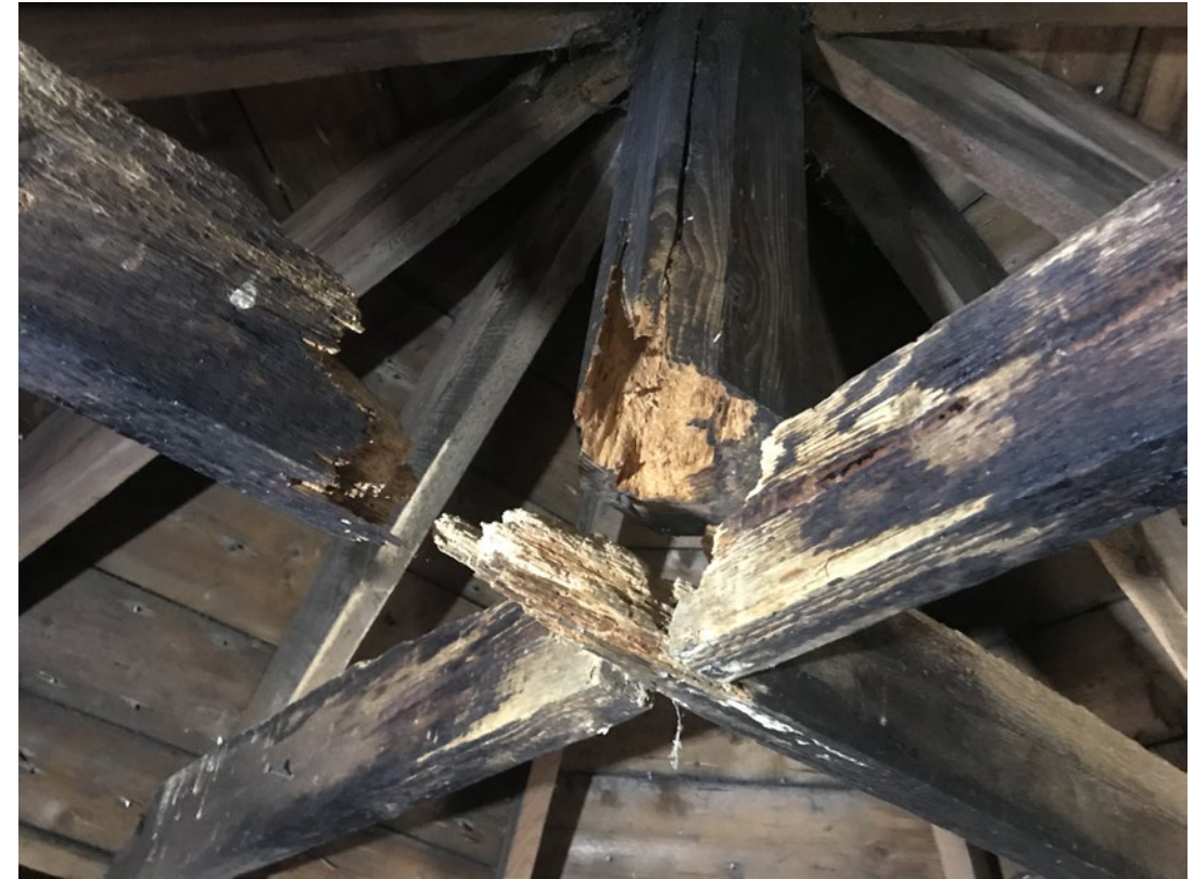
Base of the finial and support cross-ties degraded and decayed by surface/ rain water entering at the external lead covering. A repair will involve replacing the cross-ties, preparing and shuttering the finial base, and pouring structural resin into the void.
