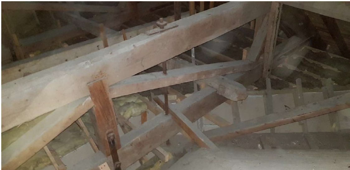
Photograph 5 – trussed members with rod present assumed to provide fixing to column below.
