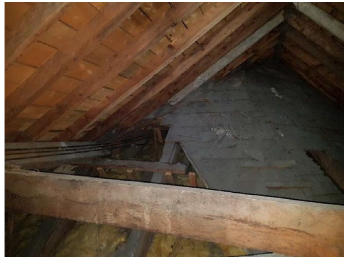
Roofspace: Remains of earlier roof structure in roofspace.
