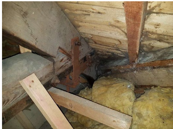
Roofspace: Some movement in main elements of timber roof structure apparent to south side of church. Metal bracing may be earlier repair to arrest structural movement and should be inspected by Structural Engineer.
