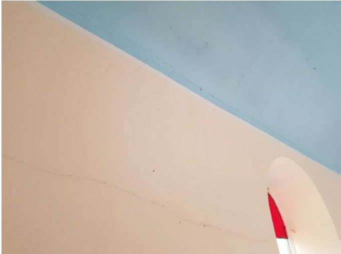
North Wall: Extensive cracking to plasterwork ceiling and walls.
