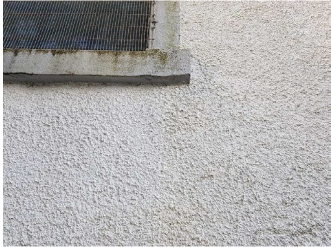
East Elevation: Cracks in harling extending down from window cill.
