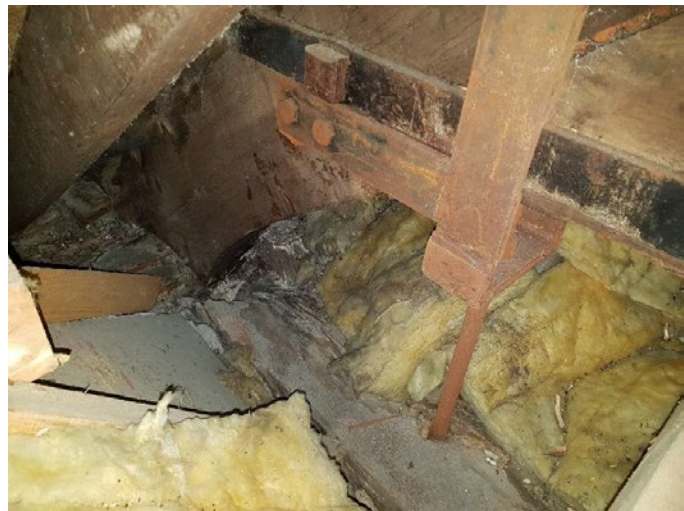
Roofspace: Staining of roof timbers and wet rot to rafters to south side of church. This is believed to be historic as it is understood repairs have now been made to replace valley flashing above.
