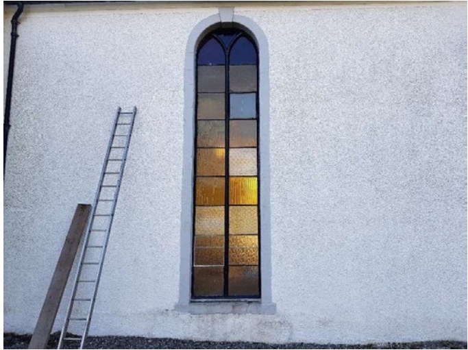
Windows: Different types and colours of glass used for previous repairs which has detracted from aesthetic appearance of windows. Assessment of the significance of the historic glass and original colour scheme needed to inform future repairs.
