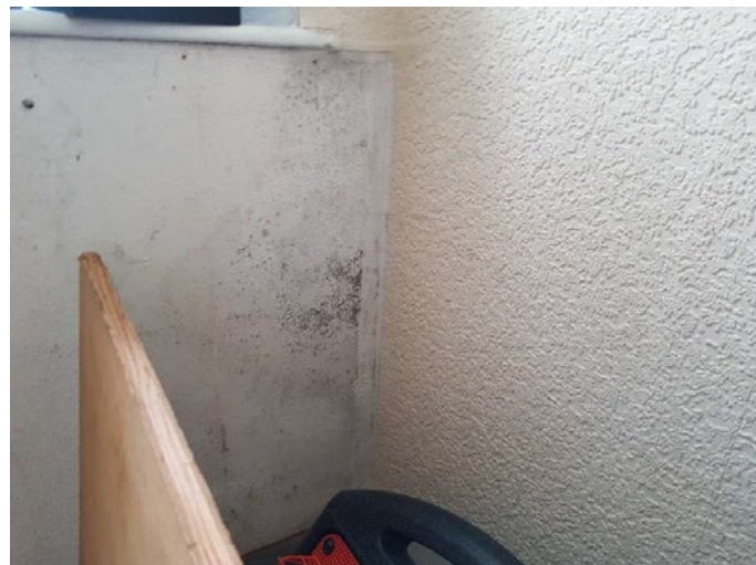
North Extension: Condensation staining and mould growth on east wall under window.
