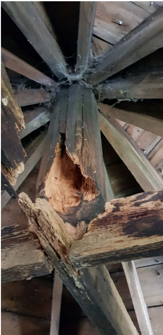
Photograph 6 – Significant section loss in cross tree members within cupola
