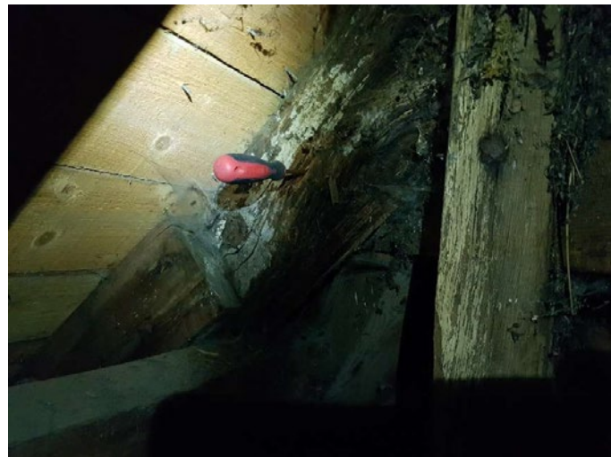
Roofspace: Rotten rafter in roofspace
