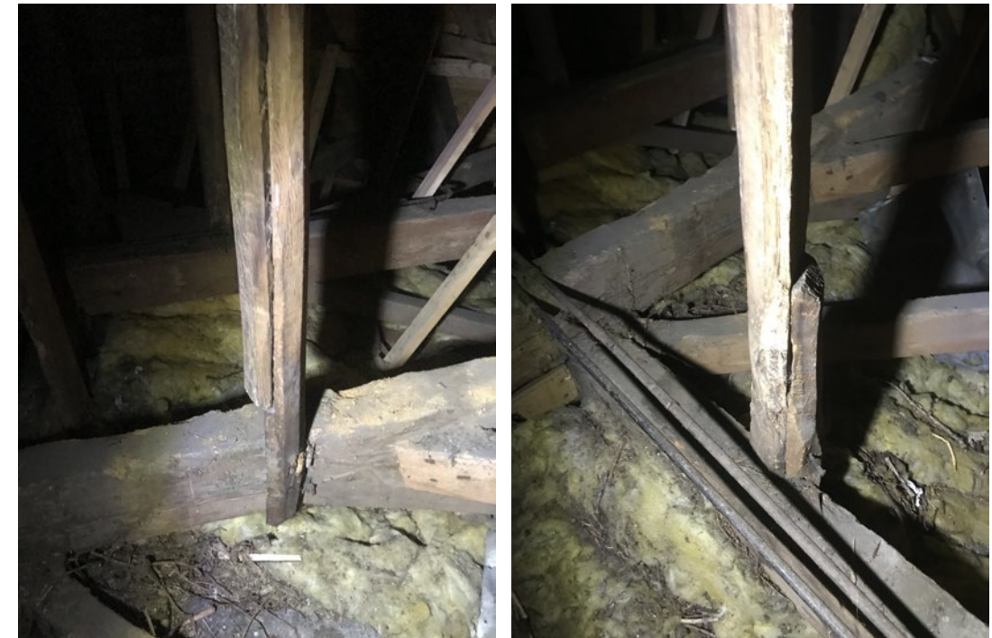
Base of oak posts: connections to principal truss collars and ties. It is recommended that these be inspected individually and strengthened with thixotropic resin injections at the oak to oak connections.
