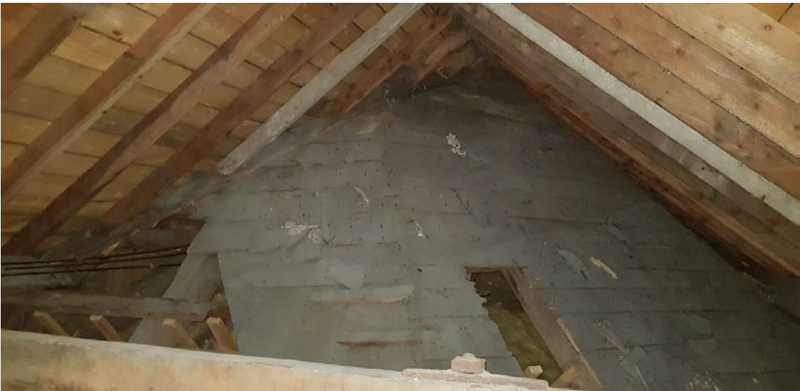
Photograph 3 – Original sarking can be seen to the octagonal roof, with the later adjoining west roof.
