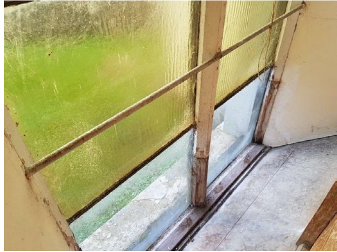
Windows: Previous timber splice repairs at base of windows. Inappropriate glazing replacements in clear glass.
