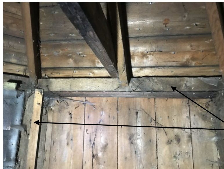
Oak Post and high-level Horizontal Tie, with roof above and sarking panel, all in good condition
