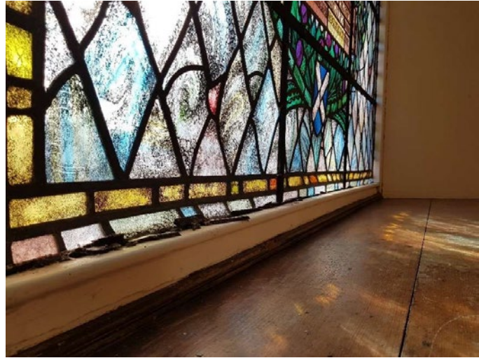
Windows: Defective putty and some distortion in lower part of leaded stained glass window.
