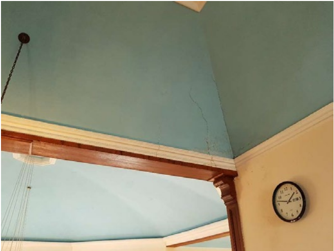
Gallery: Cracking to plaster above gallery.
