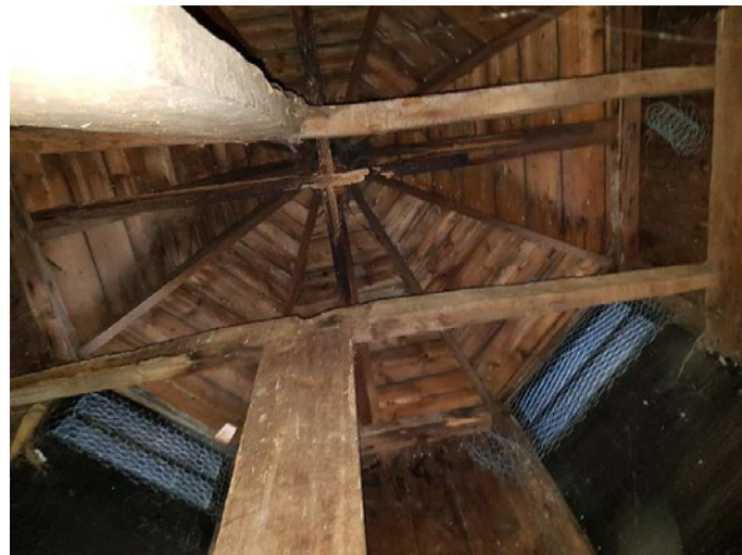
Roofspace: Broken horizontal tie to cupola.
