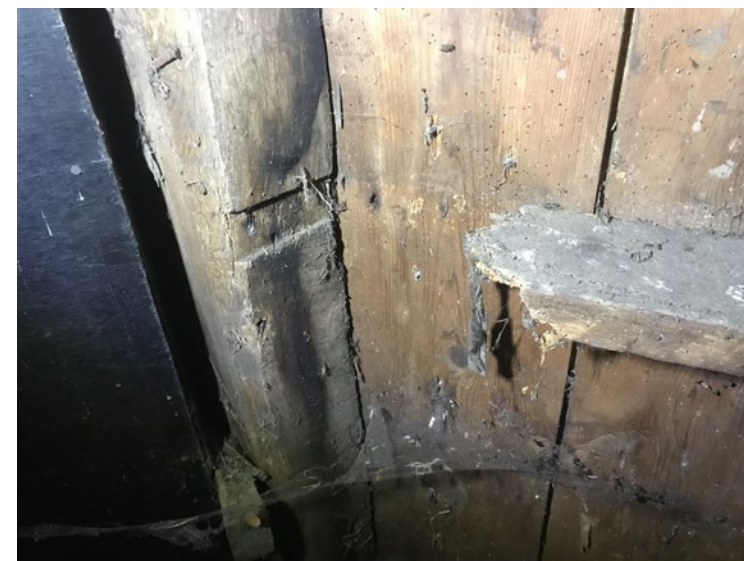
Intensely wood borer degraded softwood support member had been let-into the oak post
