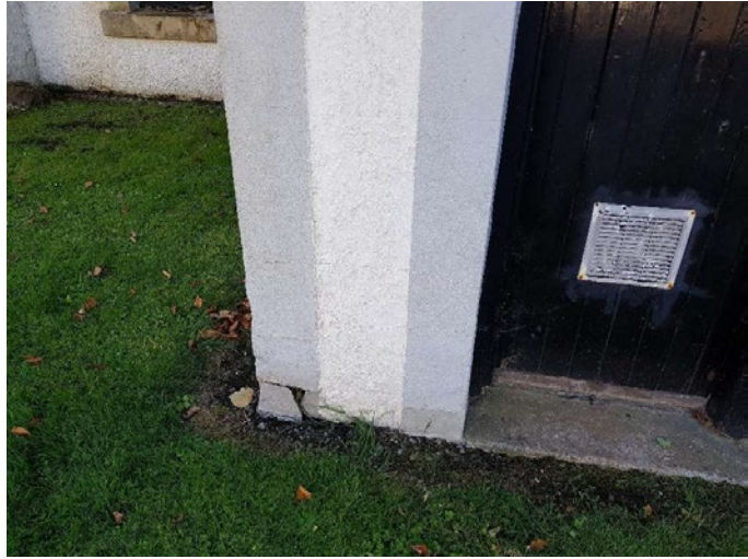
North Elevation: Cracked and spalling render at base of wall to boiler house extension to north. Plastic vent to door.
